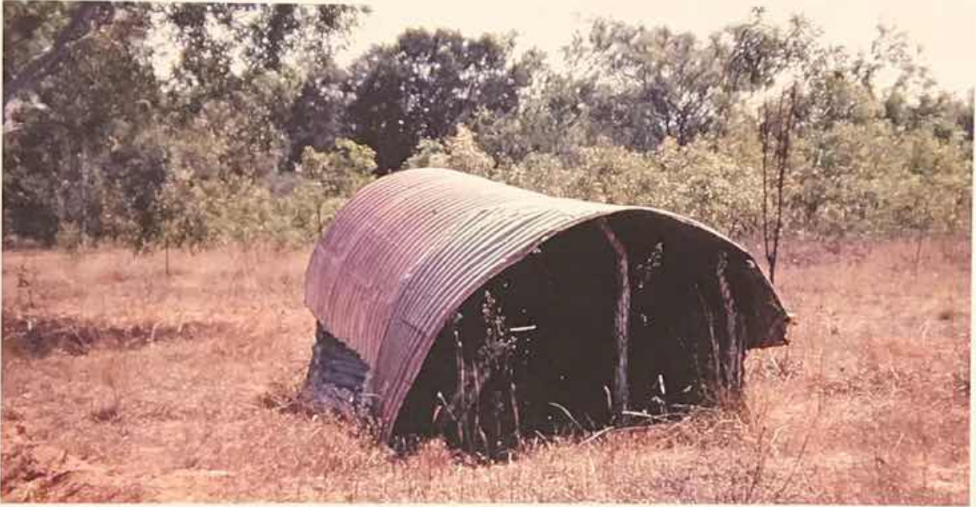
Dilapidated Metal House at Roper Bar
